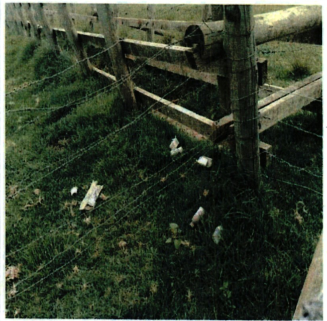
Solar Powered electric fence in Narok
