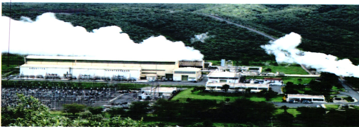
165.4MW Olkaria V Power Plant and sub-station
