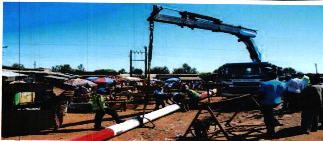
Installation of high mast in Lwanda Market
