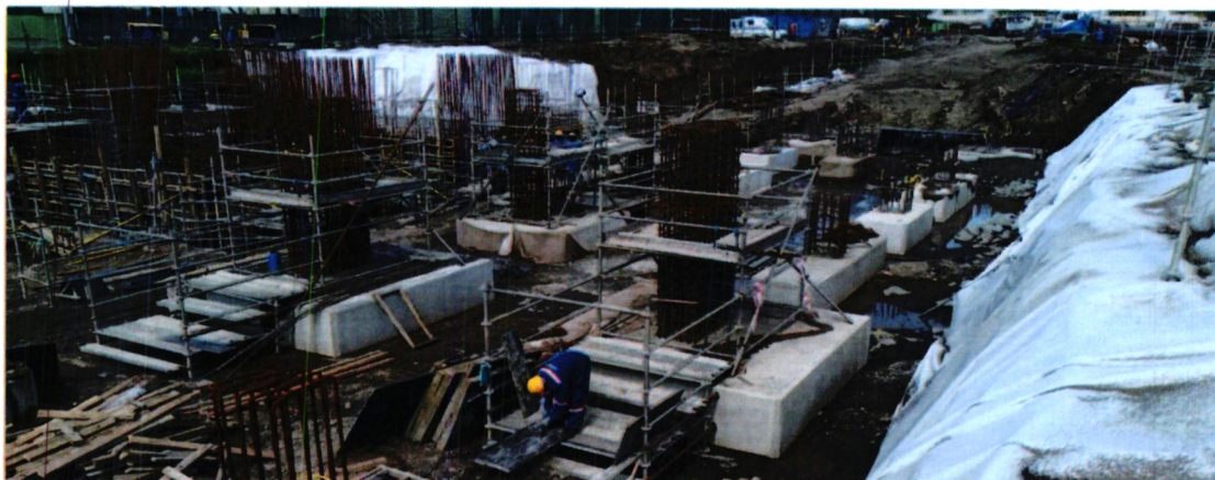
Olkaria 1 Unit 6 – Power plant substructure
