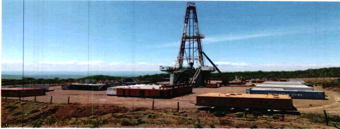
Drilling of Wells at Korosi in Baringo-Silali Geothermal Fields
