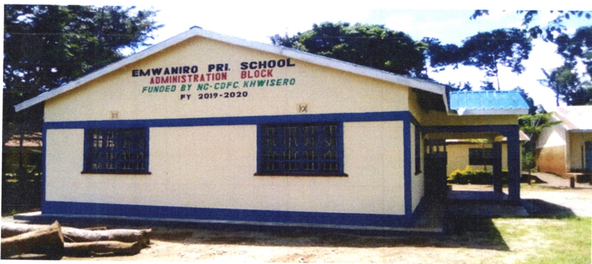
Emwaniro Primary School - Construction of an Administration block to completion. Located in Kisa Central Ward. Costed Ksh.1,800,000.
