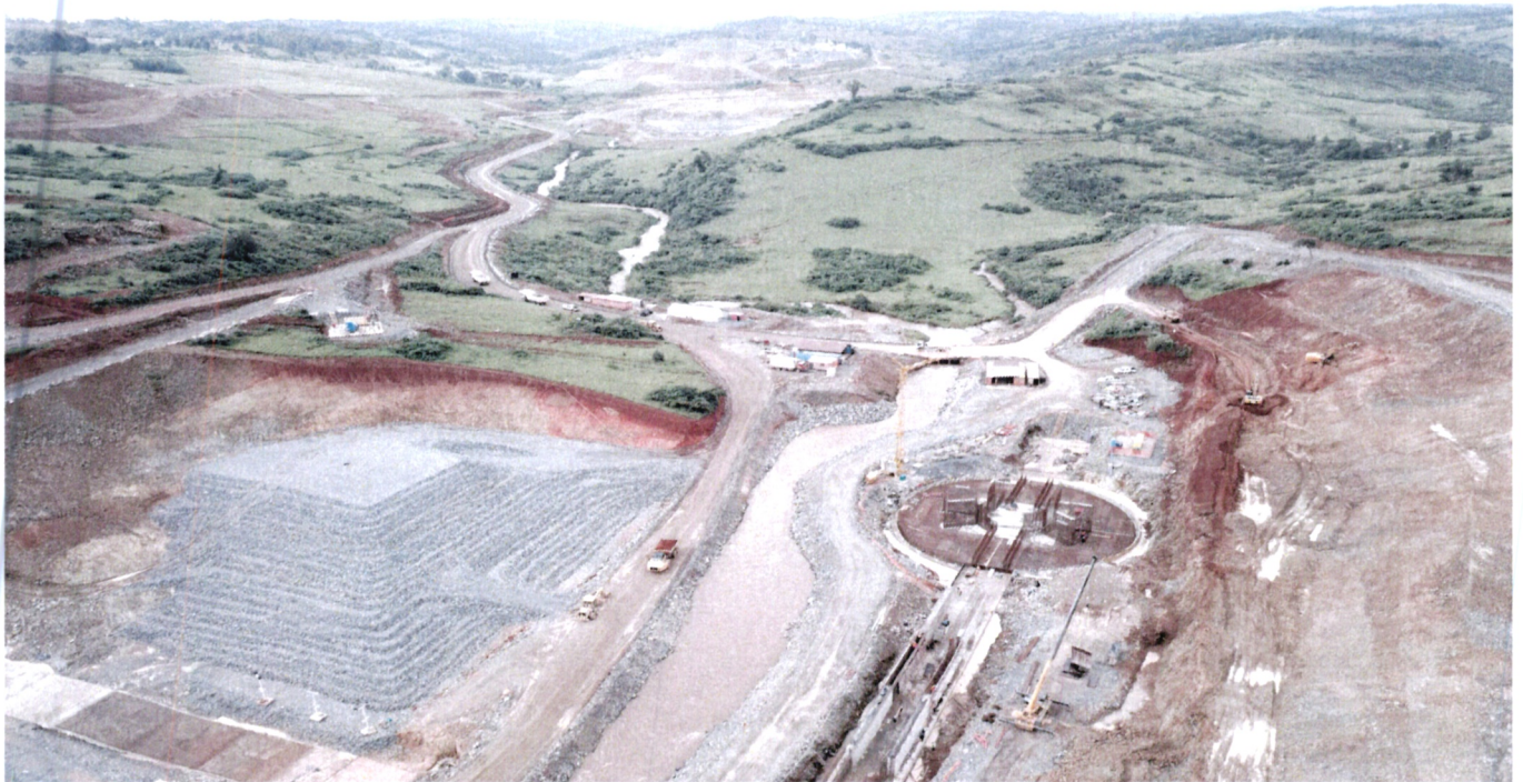
Itare Dam Water Supply Project status
