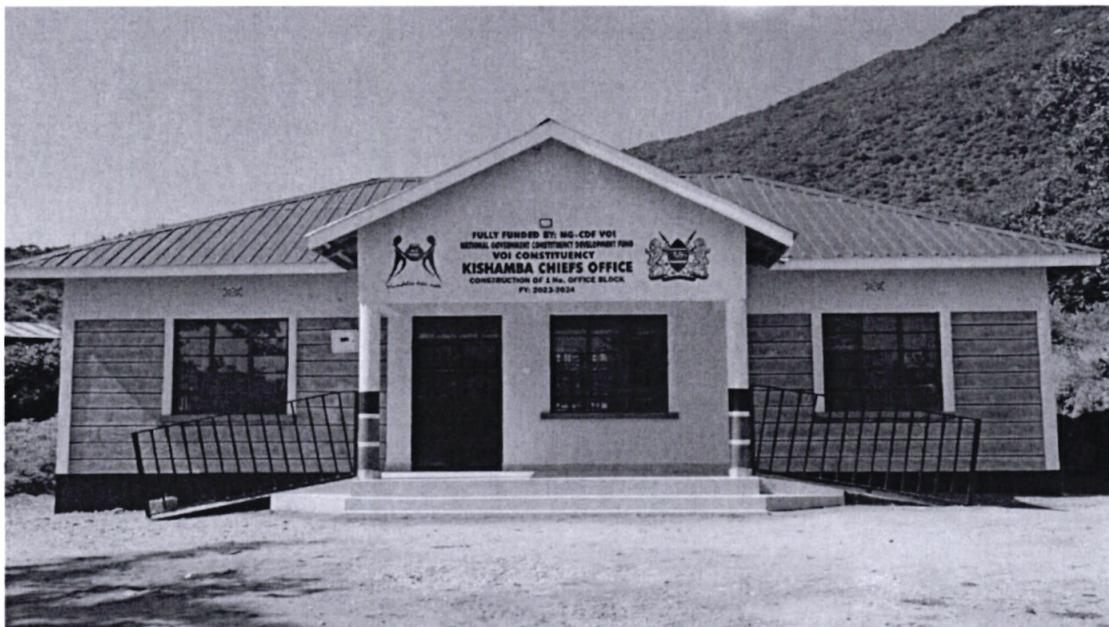
Construction to completion of Kishamba Chiefs Office
