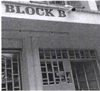
Installation of CCTV Cameras
