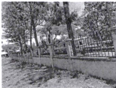
Construction of a perimeter wall
