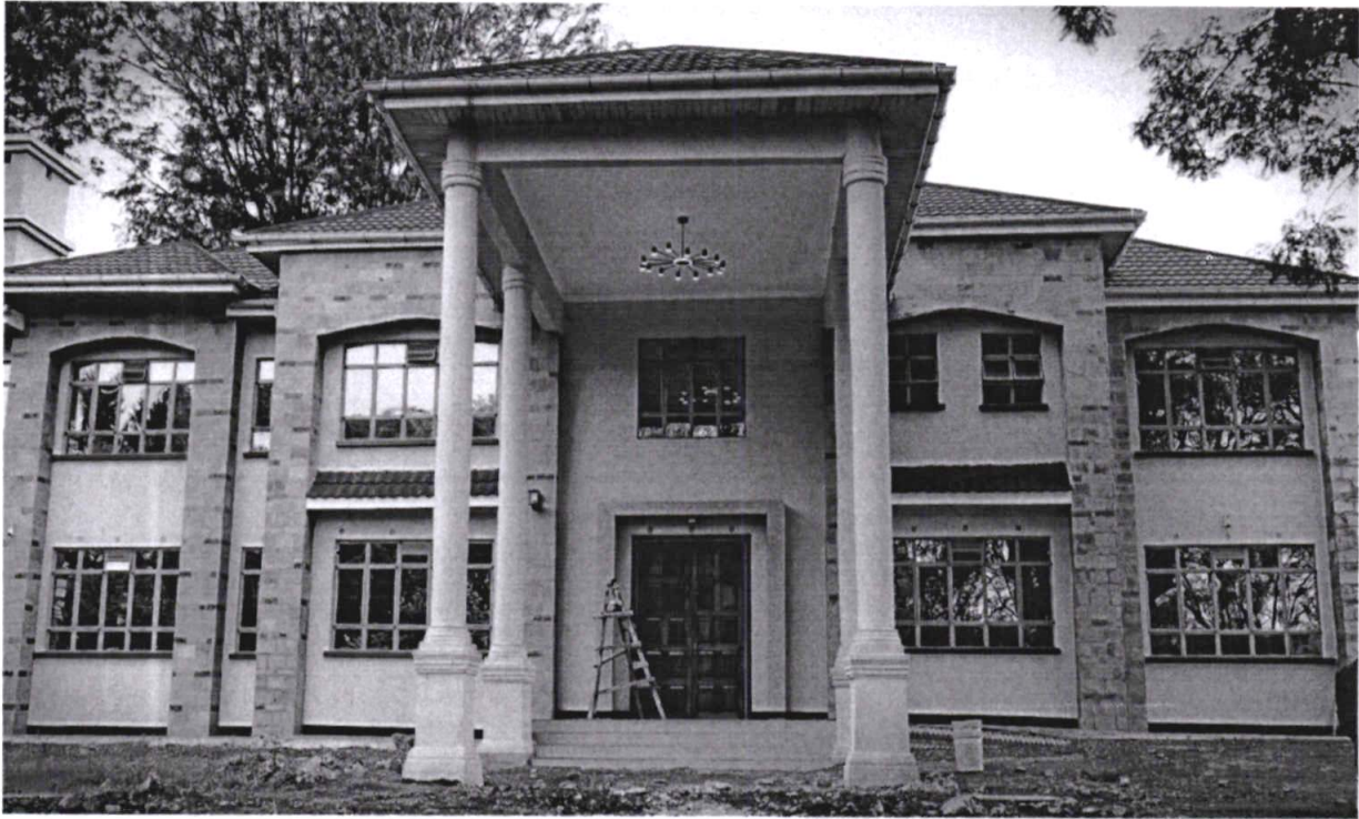
Completed construction of the official resident House for Hon. Speaker to the County Assembly
