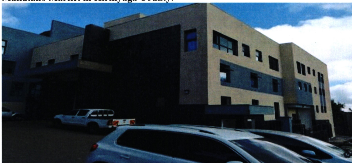
Construction of Meru County Headquarters (Meru County Investment & Development Corporation)
