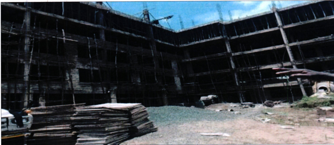
Construction of Hospital Plaza complex at Vihiga County.
