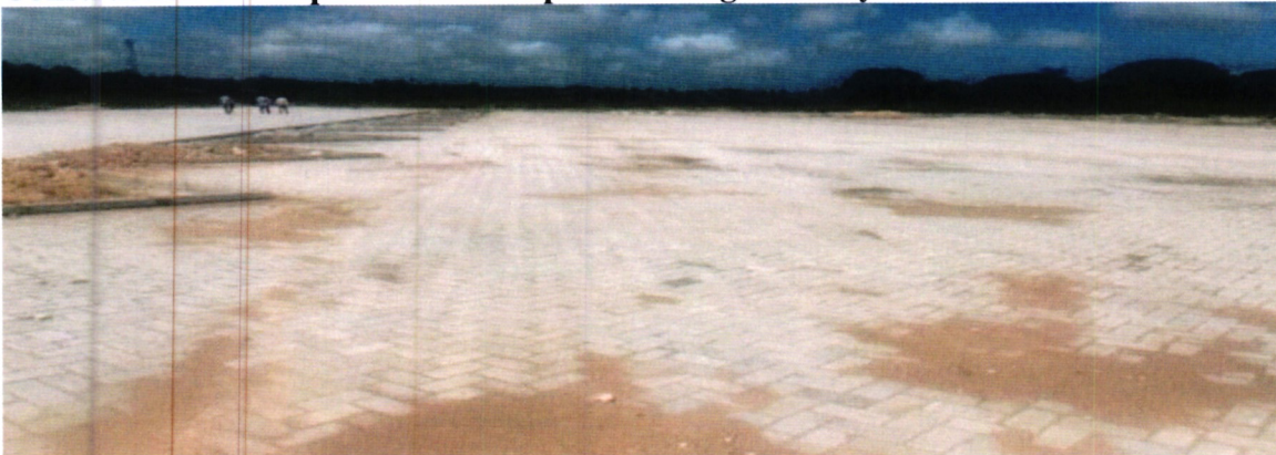
Completion of Mtwapa Bus Park in Kilifi County.
