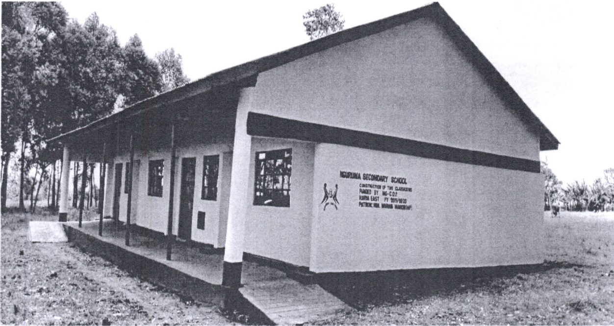
Figure 2. Nguruna Secondary school classrooms Completed in Fy 2019/2020
