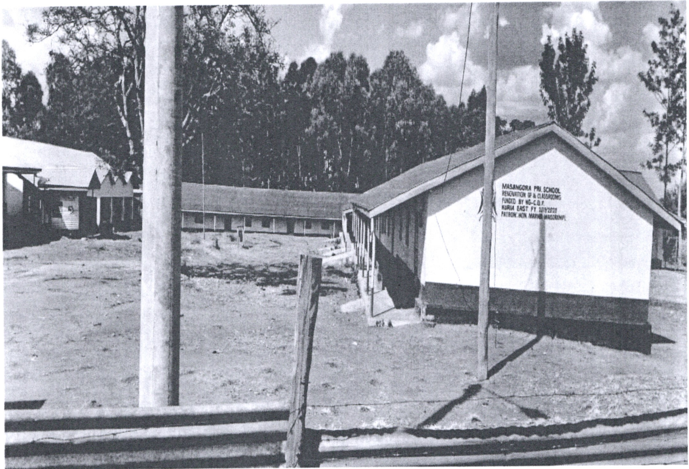
Figure 3. Masangora Primary .Renovation of fourteen classrooms and Administration Block
