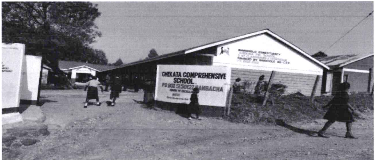
Chekata Primary School – construction of 5no. Classrooms under emergency funds in Bunyala West Ward, complete and handed over
