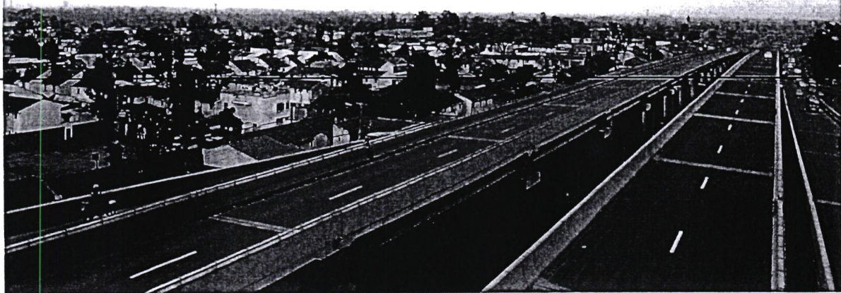
The road section at Km 4+500 (near Kangundo Road viaduct)
