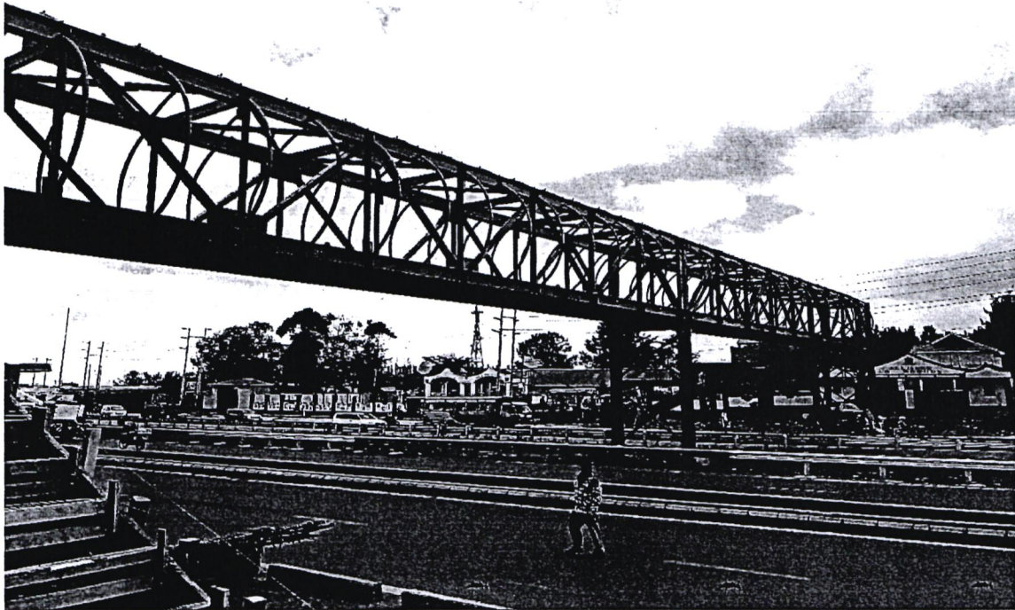
The footbridge under construction at Km 1+890 (near Access to Kiamaiko)
