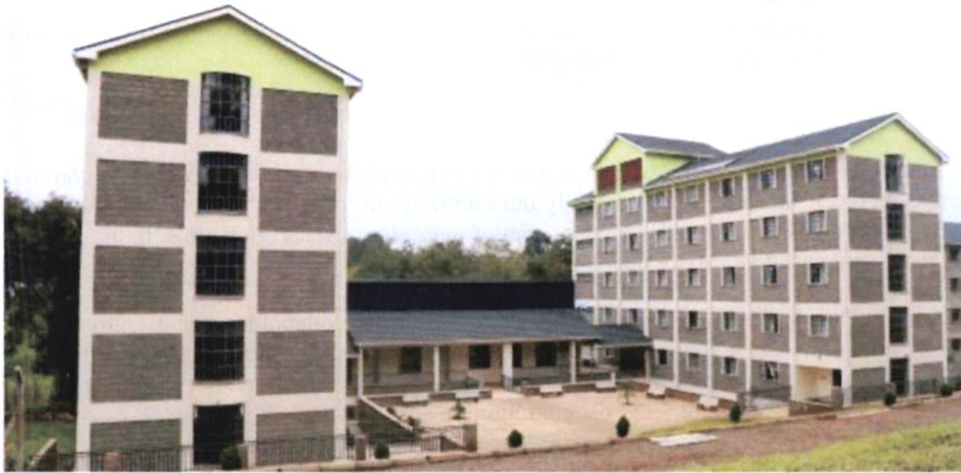
Figure10: Front view of the capitalised Hostel Block Phase 3
