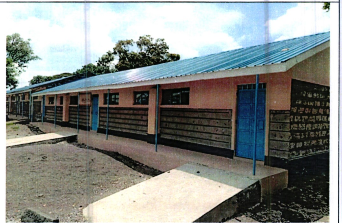
Mwariki Primary Primary School - Construction of Two classrooms (Complete and Furnished)
