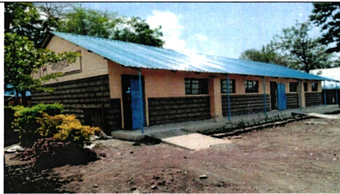
Eileen Ngochoch Primary School - Construction of Two classrooms (Complete and Furnished)
