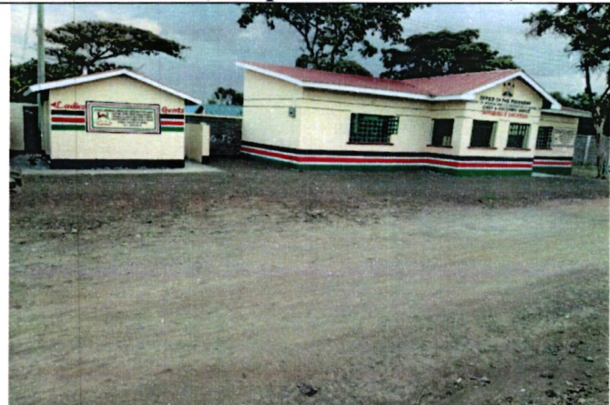
Mwariki Chief/ Ass. Chief Office - Construction of 3 roomed office & Public Toilet(Complete)
