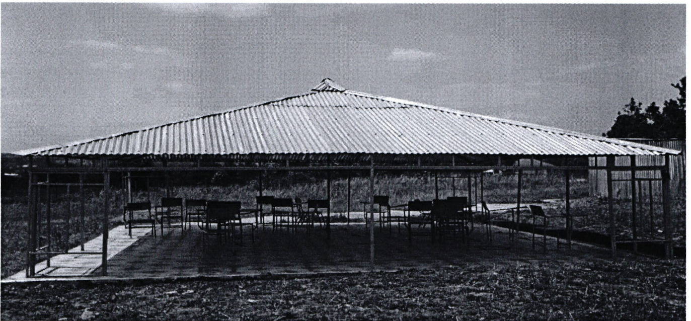
More advance temporary leaning make-shift
