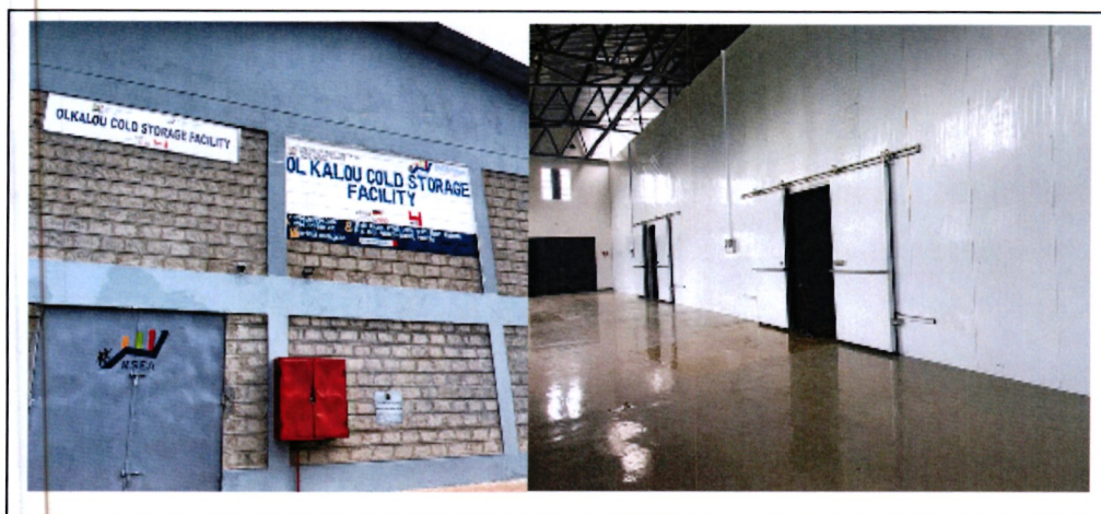
Picture 7: The Ol Kalou Cold Storage Facility Not in Use
