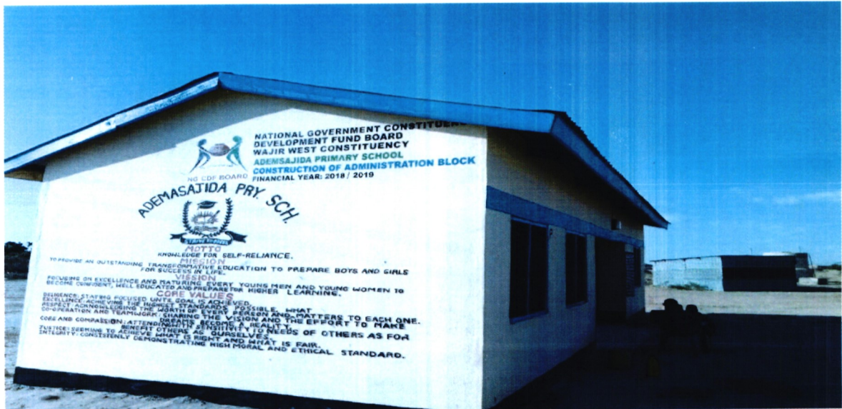
An administration Block at Ademasajida Primary School in Wajir West Constituency implemented during the FY 2019/20120
