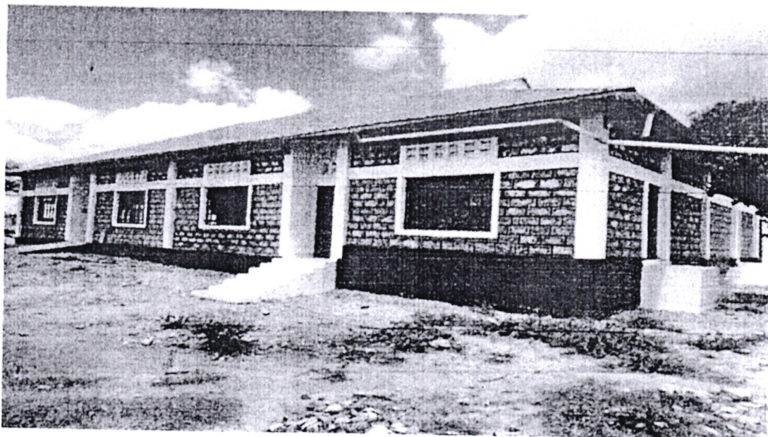
Mwalewa Girls Secondary school multi-purpose dining hall with annex kitchen
