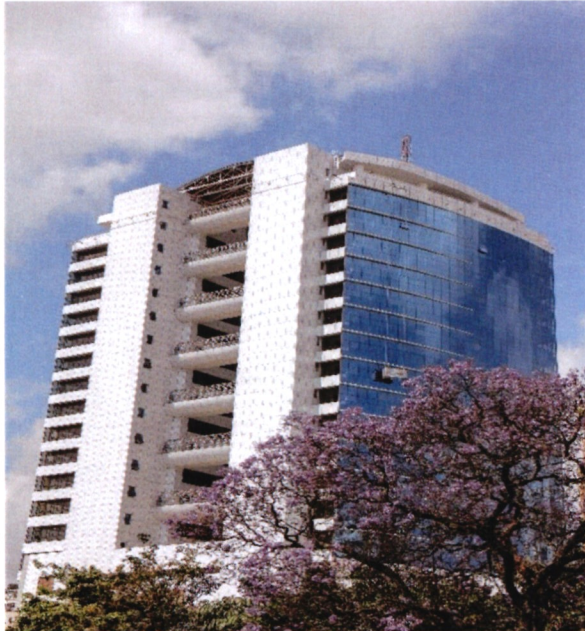
Hazina Trade Centre in Nairobi was completed this year and is now ready for occupation.
