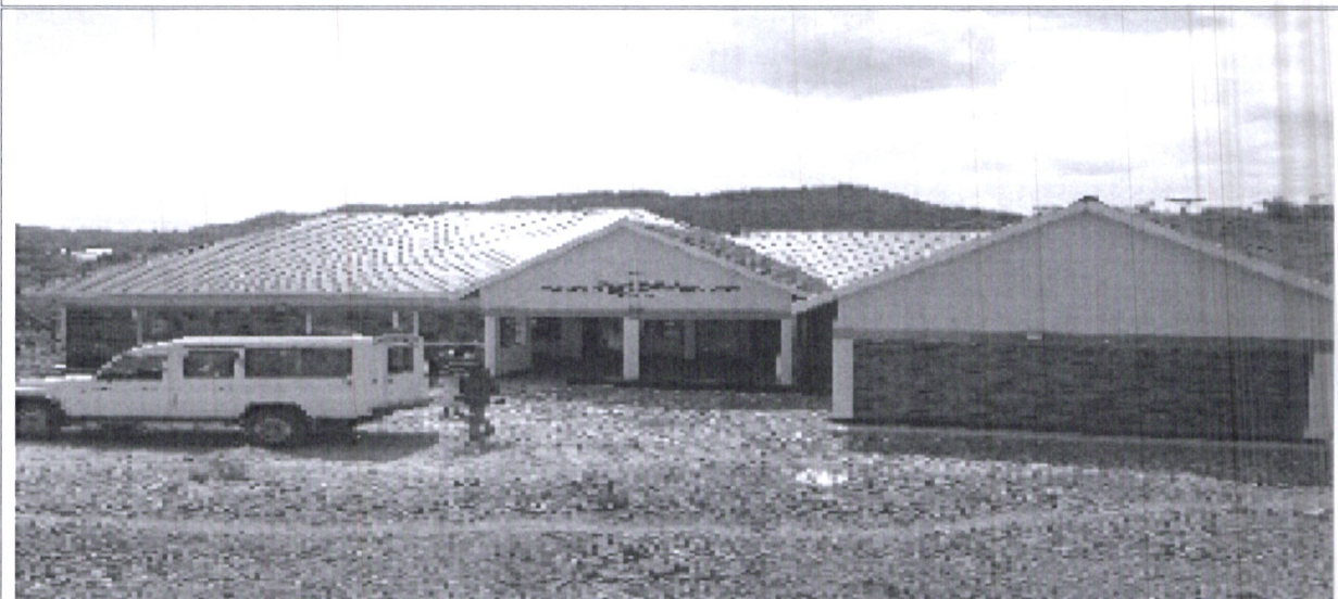
Turkana North NGCDF Office Construction of NGCDF office
