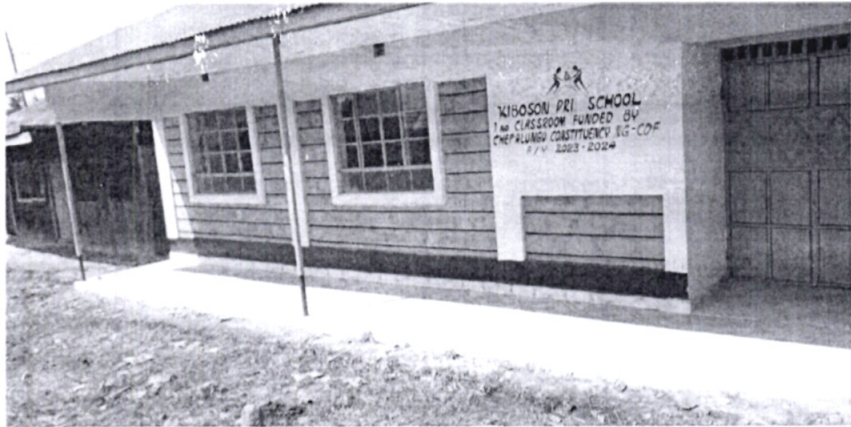
Project 1: Kiboson Primary School (construction of one classroom FY 2023/2024)
