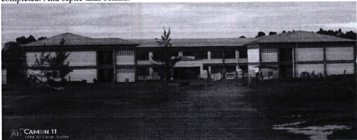
Block 1A Mechanical workshop Complex given a facelift (Above)
