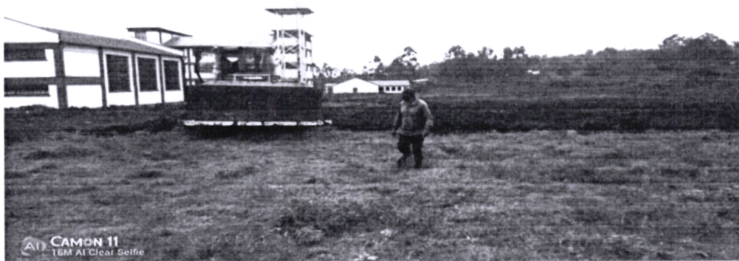
Drainage system preparation above.
