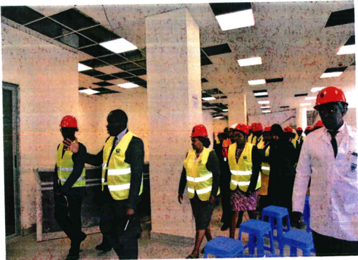
Inspecting construction works at the East African Centre for Urology and Nephrology
