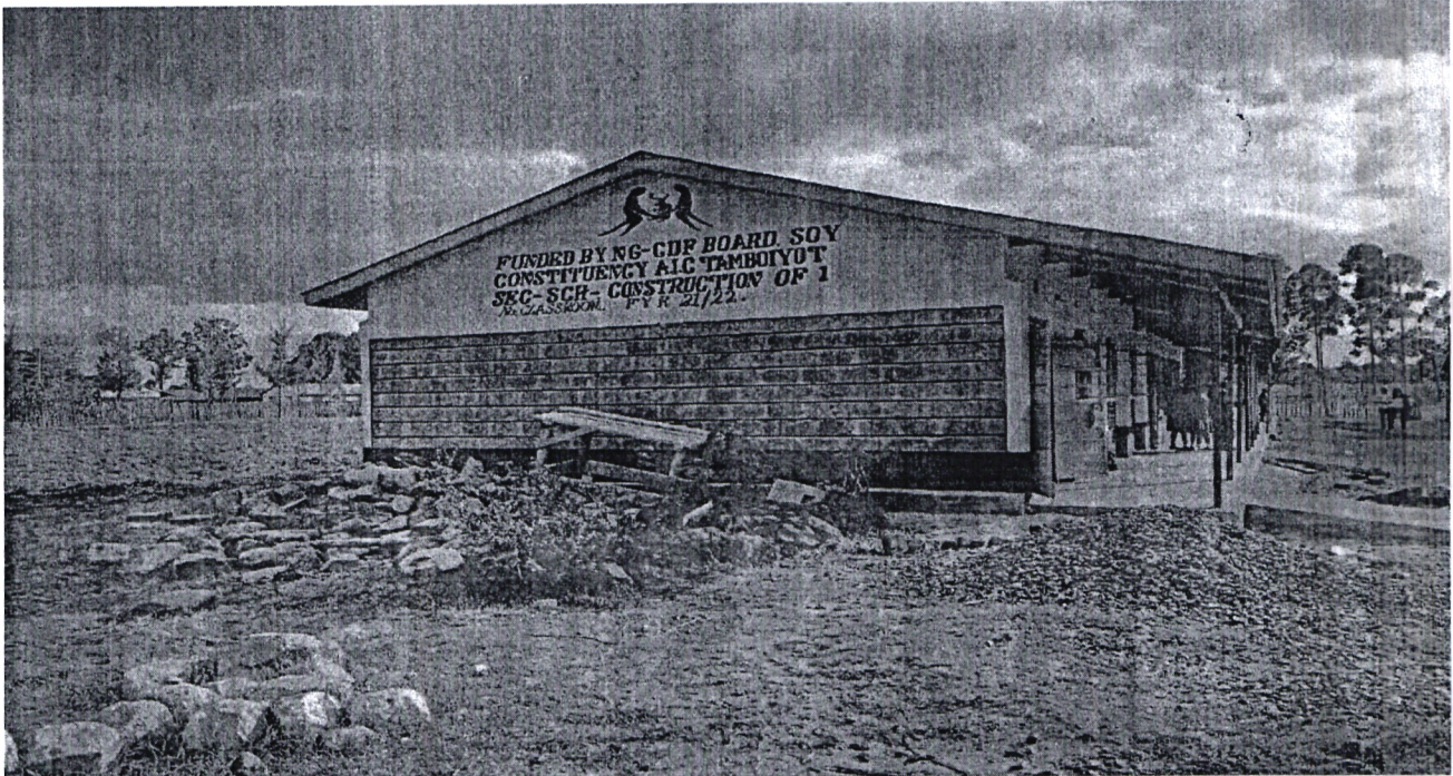
Photo1. AIC Tamboiyot Secondary School construction of 1 classroom. Impact: Enhanced conducive learning environment.
