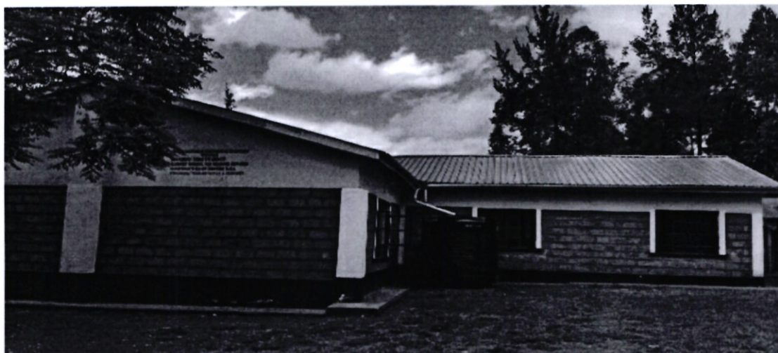
Eldoret school for the hearing impaired -construction of dining hall
