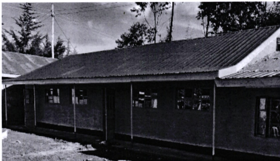
Chepkero Primary-construction of classroom
