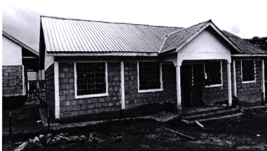
Rurigi Secondary- Construction of Admistration Block
