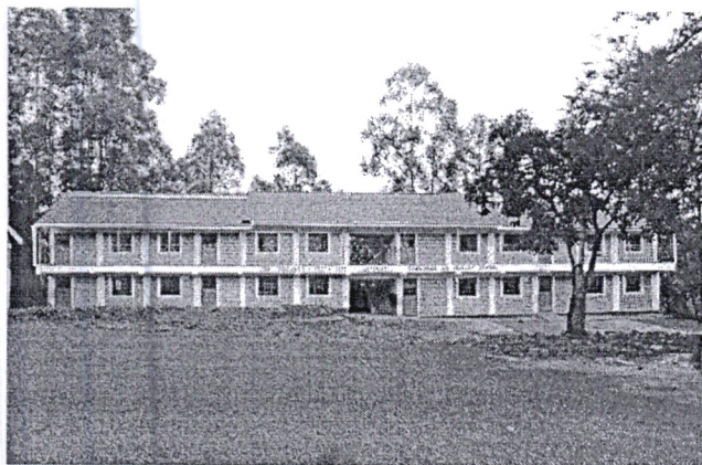
Eregi Mixed Primary School-Construction of 8No. Storey Classrooms
