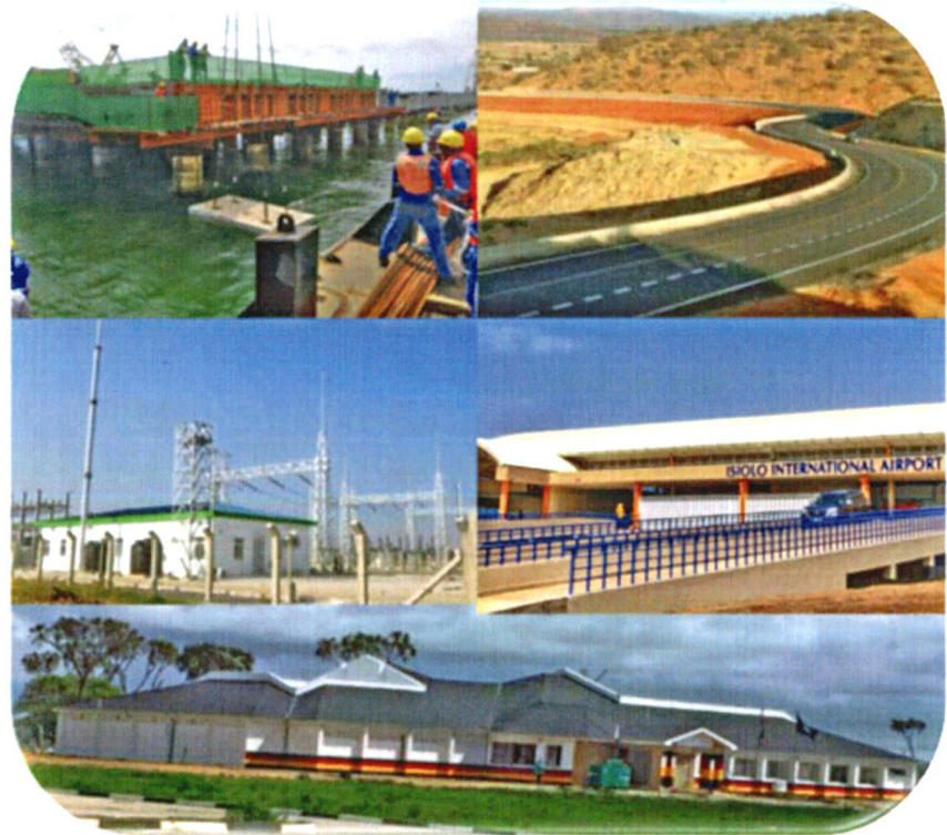
Figure 21: Ongoing Lapsset Project
