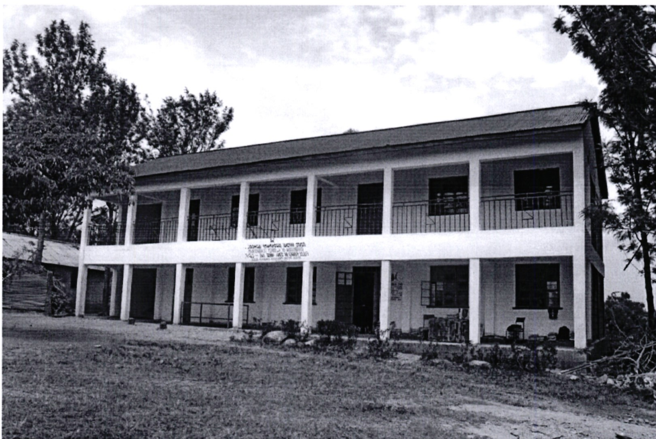
BONDO NYIRONGE PRIMARY SCHOOL 4 STOREY CLASSROOMS
