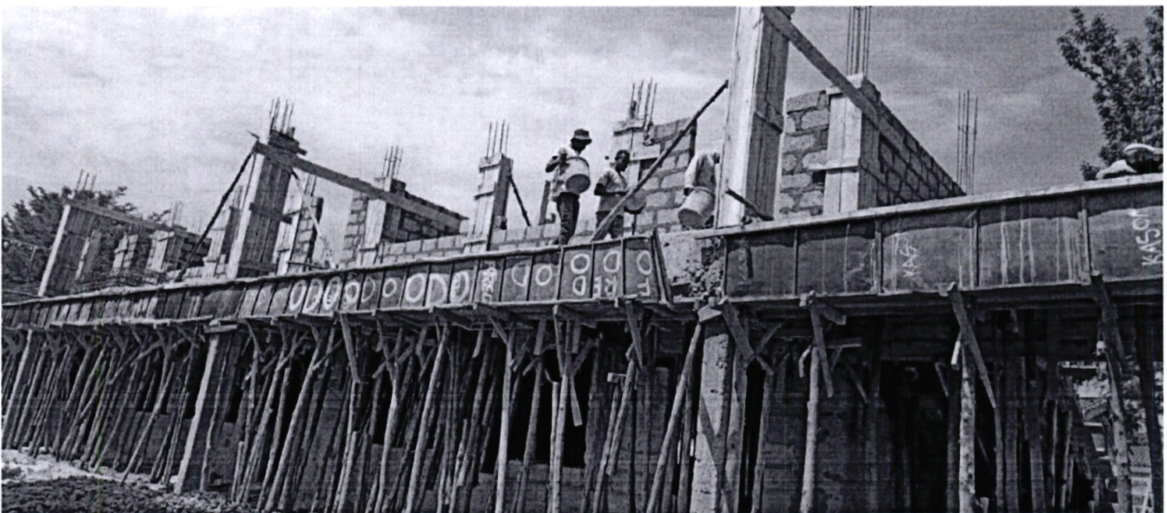
On-going construction of 4- storey 12 lecture halls
