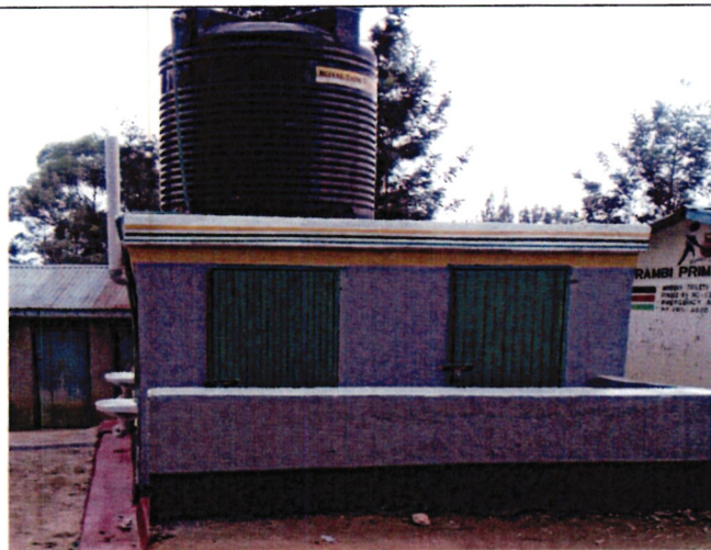
Ablution facility for St. Basil Lurambi Primary School, Kakamega County.
