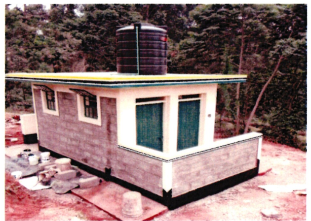
Ablution facility for Kiiri Secondary School, Muranga Country.
