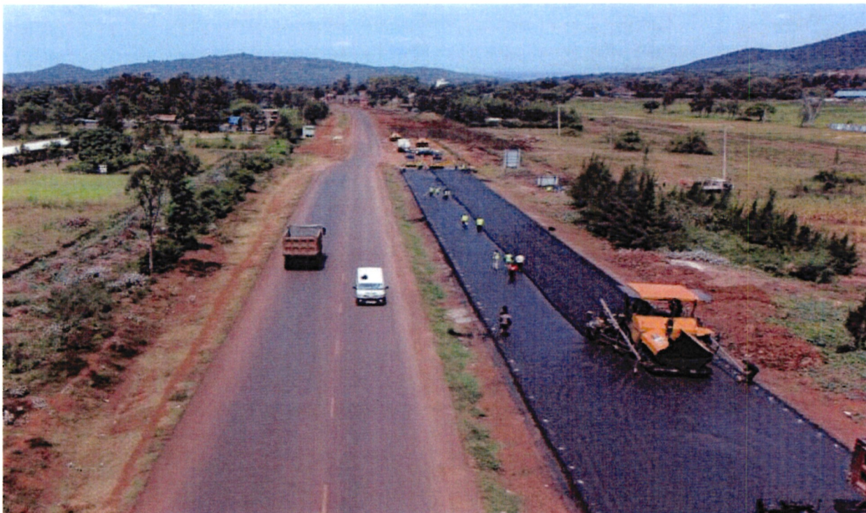
Picture 1: Section of Kenol-Sagana-Marua under construction
