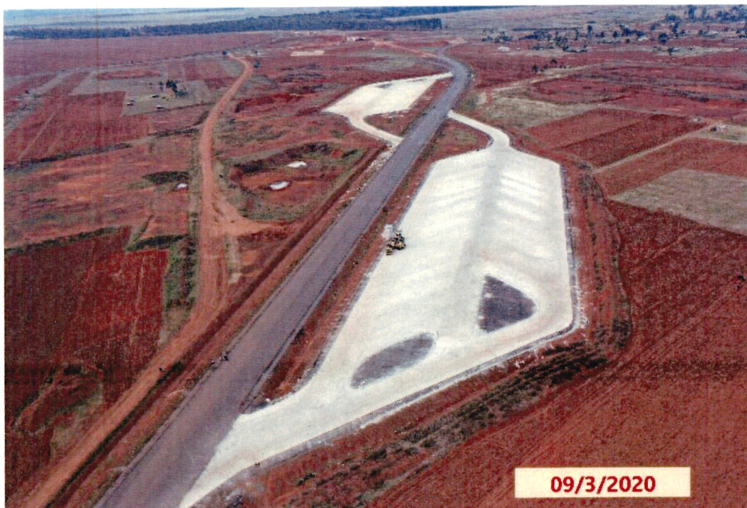
Figure 2: Aerial view of completed Truck parking bays at Leseru (Km 30+600)
