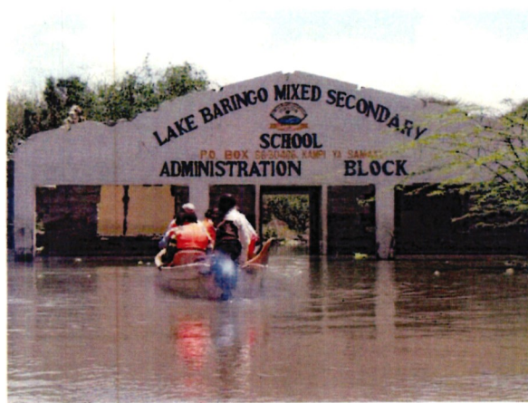
Flooded administration block and classrooms at Lake Baringo Mixed Secondary Schools, Baringo County.
