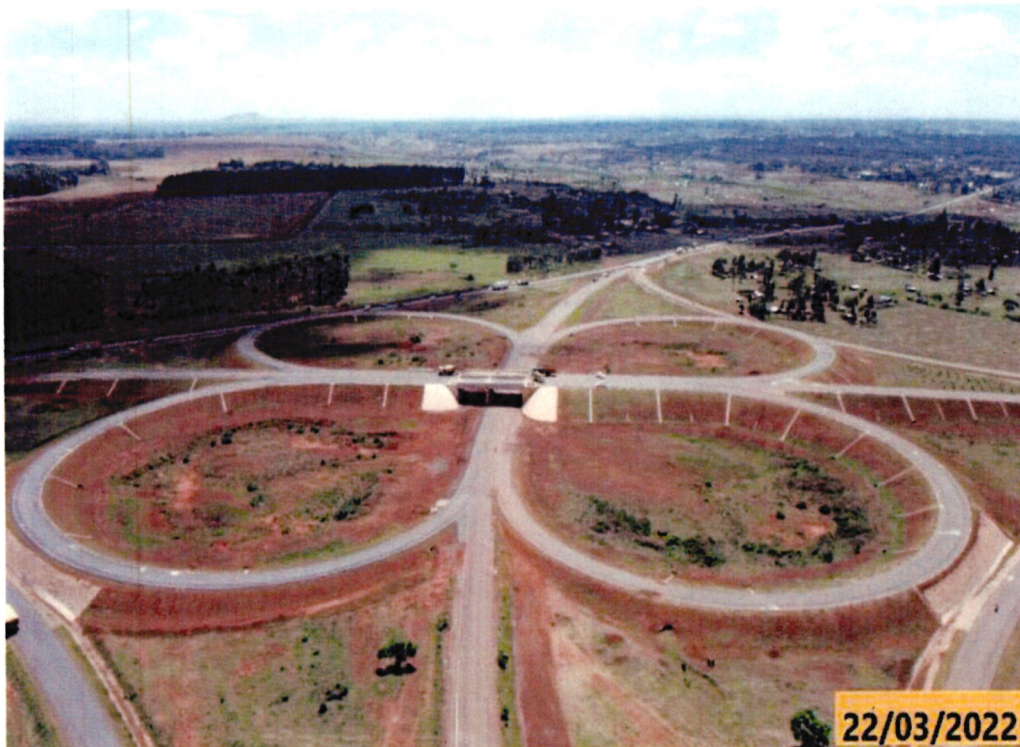
Figure 1: An aerial view of Leseru Interchange at km 31+200
