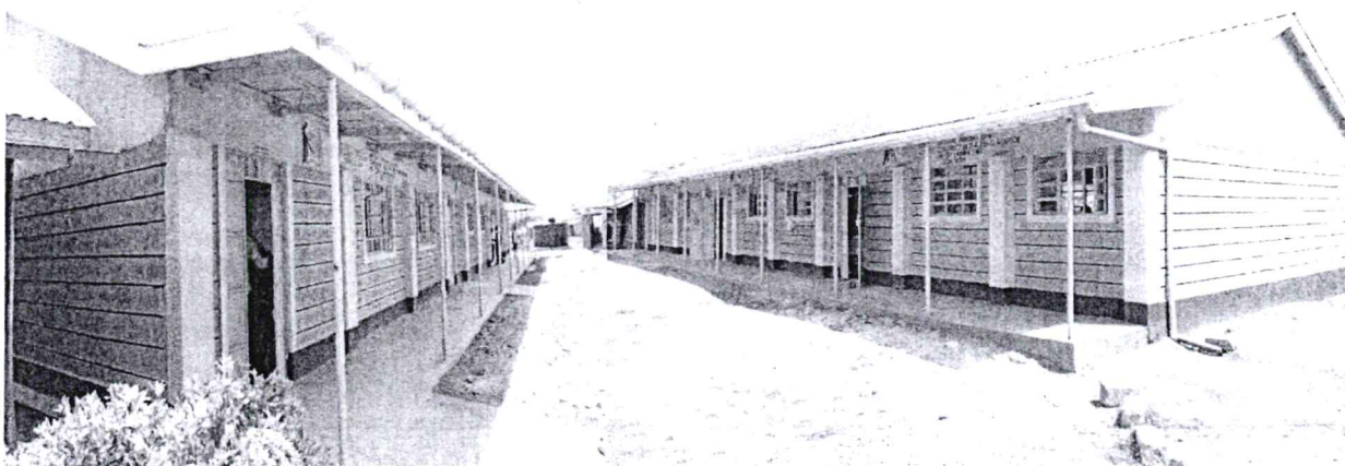
WITHARE PRIMARY SCHOOL- CONSTRUCTION OF 3 CLASSROOMS
