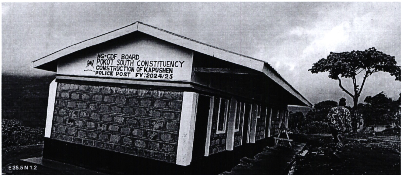
Kapushen Police Post. Construction of single Police House
