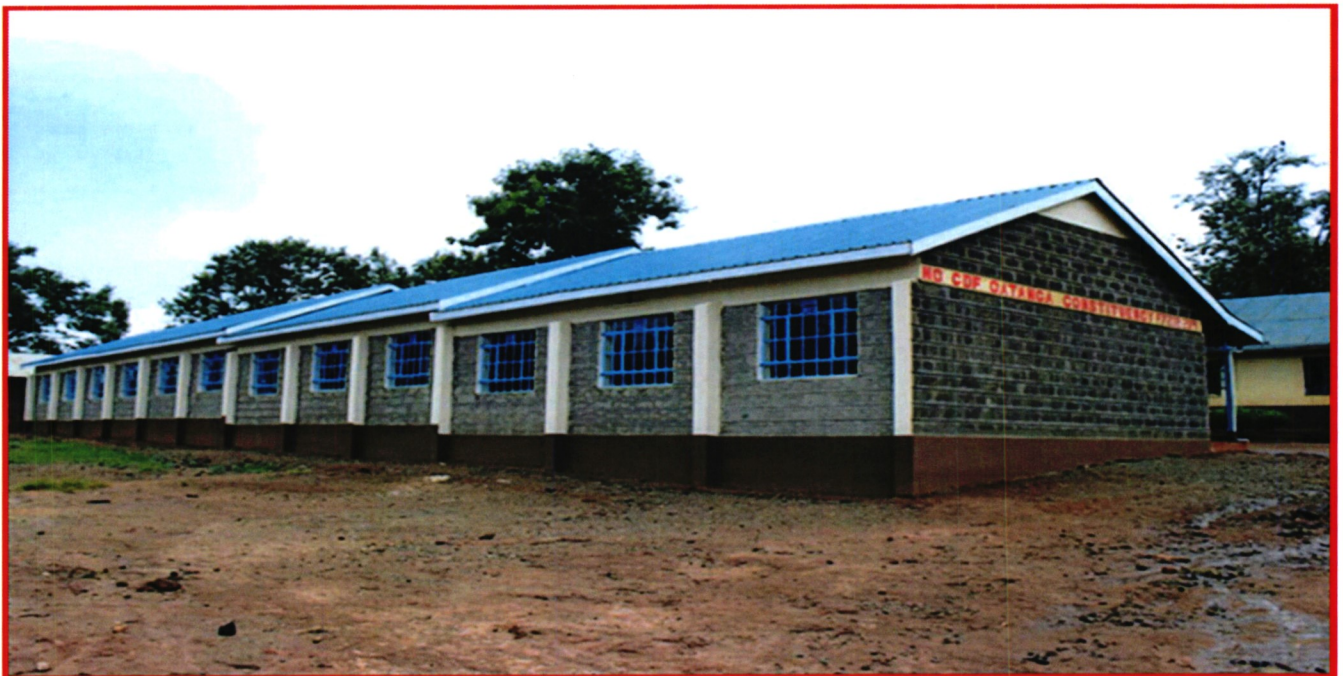
Construction of four Standard Classroom at Ngatho Primary School (The project expected to provide a 160 pupil learning space each year and 120 pupils learning space where COVID-19 is concern)
