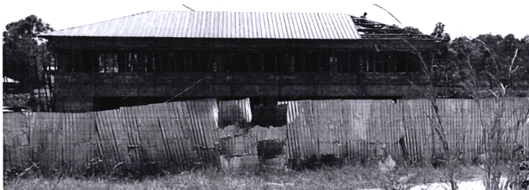
The Hospitality Complex funded by AfDB nearing completion (above)
