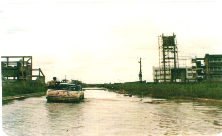
A construction site photo of KLB headquarters in South C taken on May 12, 1989.
