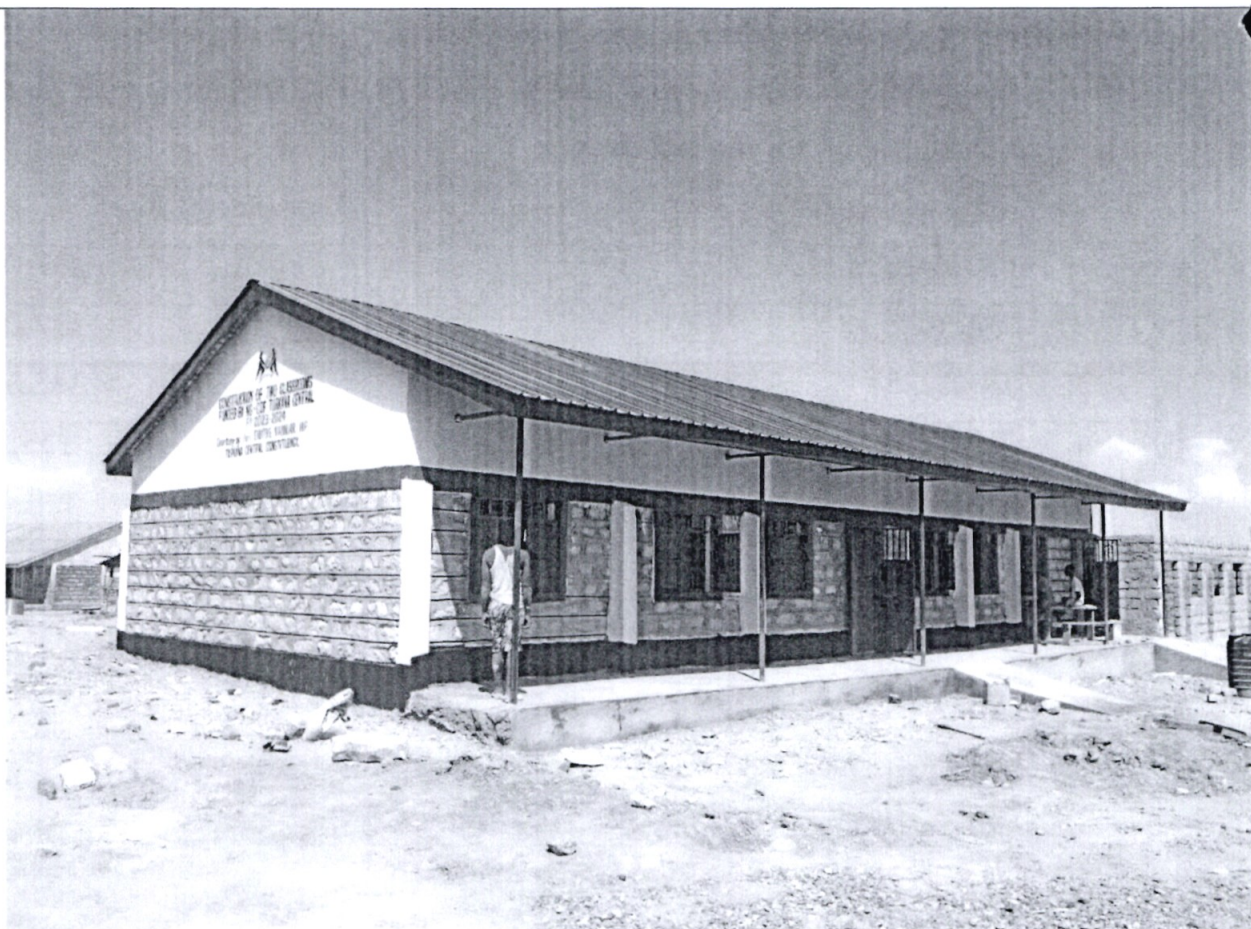
Figure 1- Kerio Primary School - Construction of JSS Classrooms
