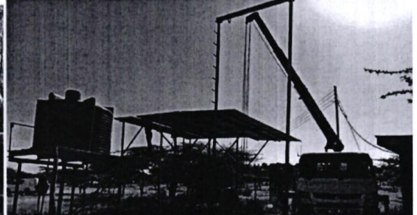
Rehabilitation of Naiperere 2 borehole, Laikipia
