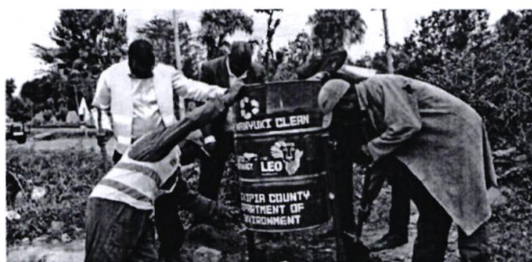
Urban Centre Waste Management - bin installation
