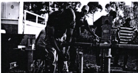
Rehabilitation of Munyu Borehole, Marmanet Ward
