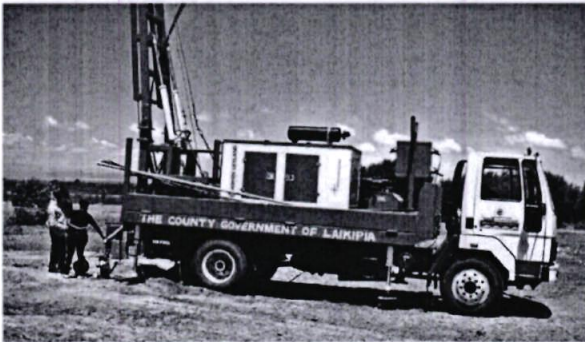
Borehole Drilling - CAIP Rumuruti Ward
