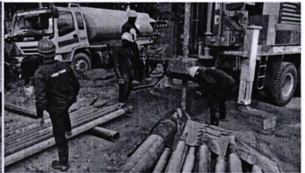
Borehole Drilling - CAIP Rumuruti Ward
