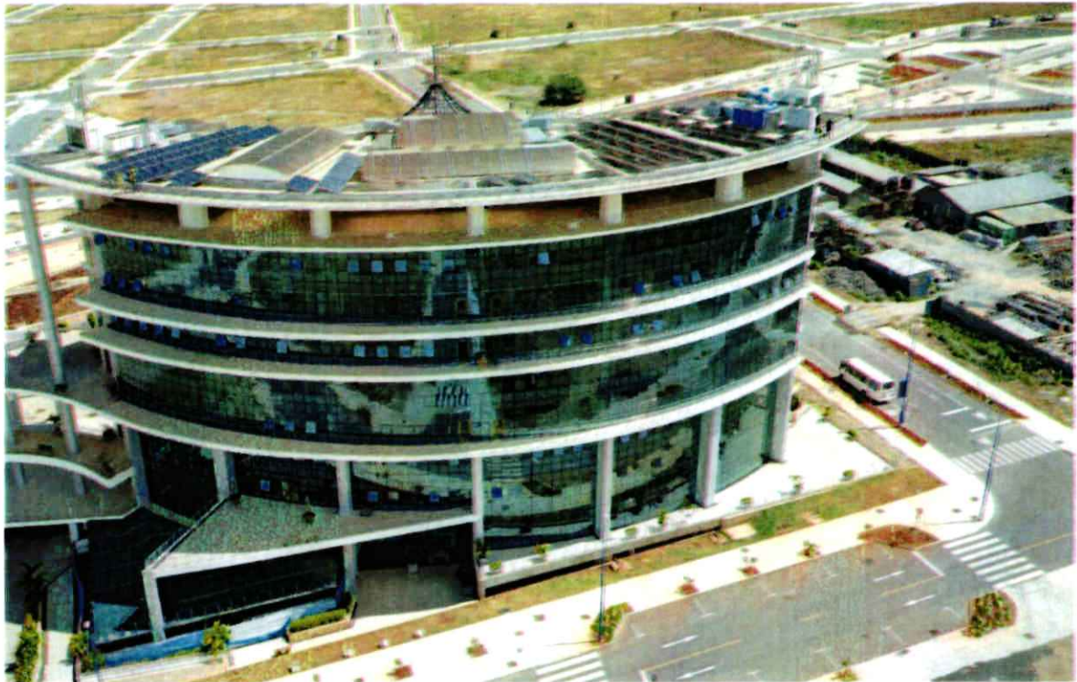
Conference Facility Superstructure Completion during the Financial Year
