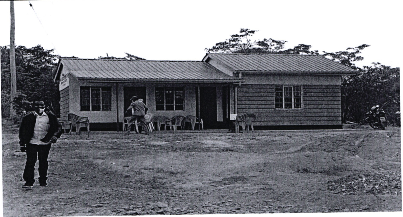
Fig. 1.2: Miau Assistant Chiefs. Construction of Assistant Chiefs Office
