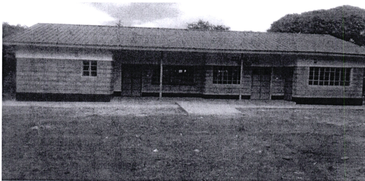
Fig. 1.1: Kiteta Chiefs Offices. Construction of Chiefs Office
