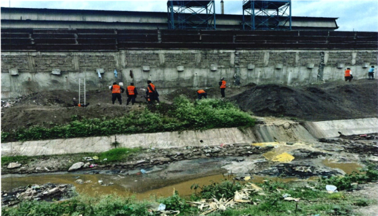
Figure 6. A sewer line operated by MAVWASCO next to Apex Steel Company in Kitengela
