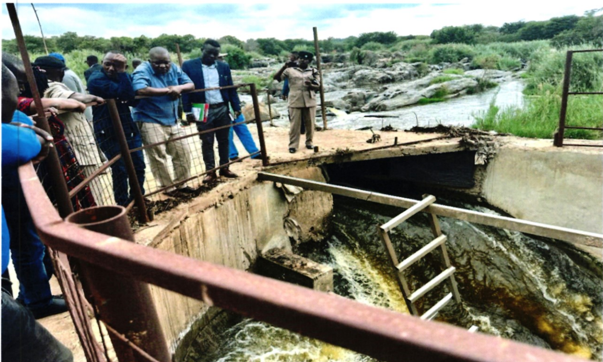
Figure 8. Members of the Public Petitions Committee inspecting the dam project along River Athi, at Kiukuuni Village in Mwala Constituency
