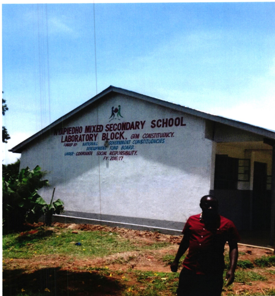
LABORATORY BLOCK AT NYAPIEDHO MIXED SECONDARY SCHOOL IN WEST GEM WARD.
