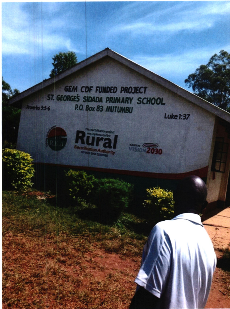
CONSTRUCTION OF CLASSROOMS AT SIDADA PRIMARY SCHOOL IN NORTH GEM WARD FUNDED BY GEM NG-CDF
