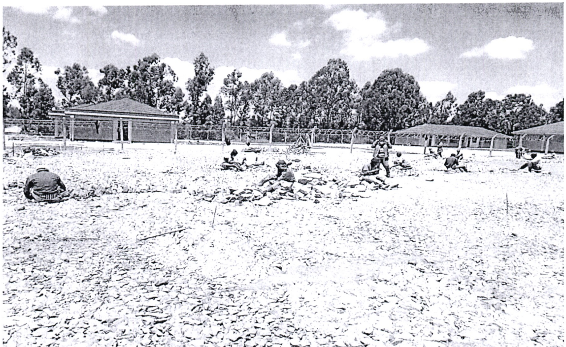
Fig 9: Hardcore hand Packing for main Car Park
