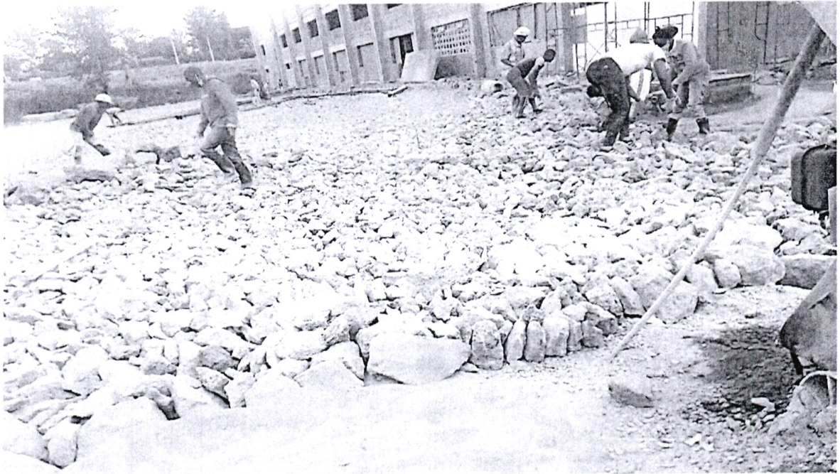
Fig 15: Hard-core hand packing of the Public parking
