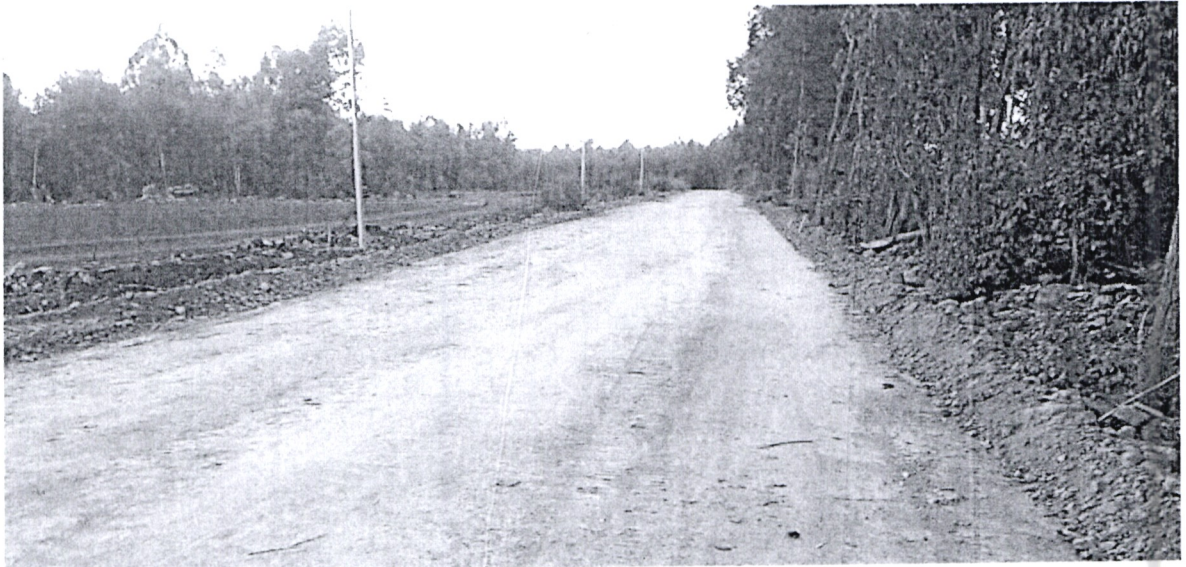
Fig 5: 3.4Km Marram track
