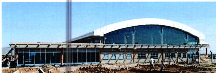
Isiolo Terminal Building 90% complete
