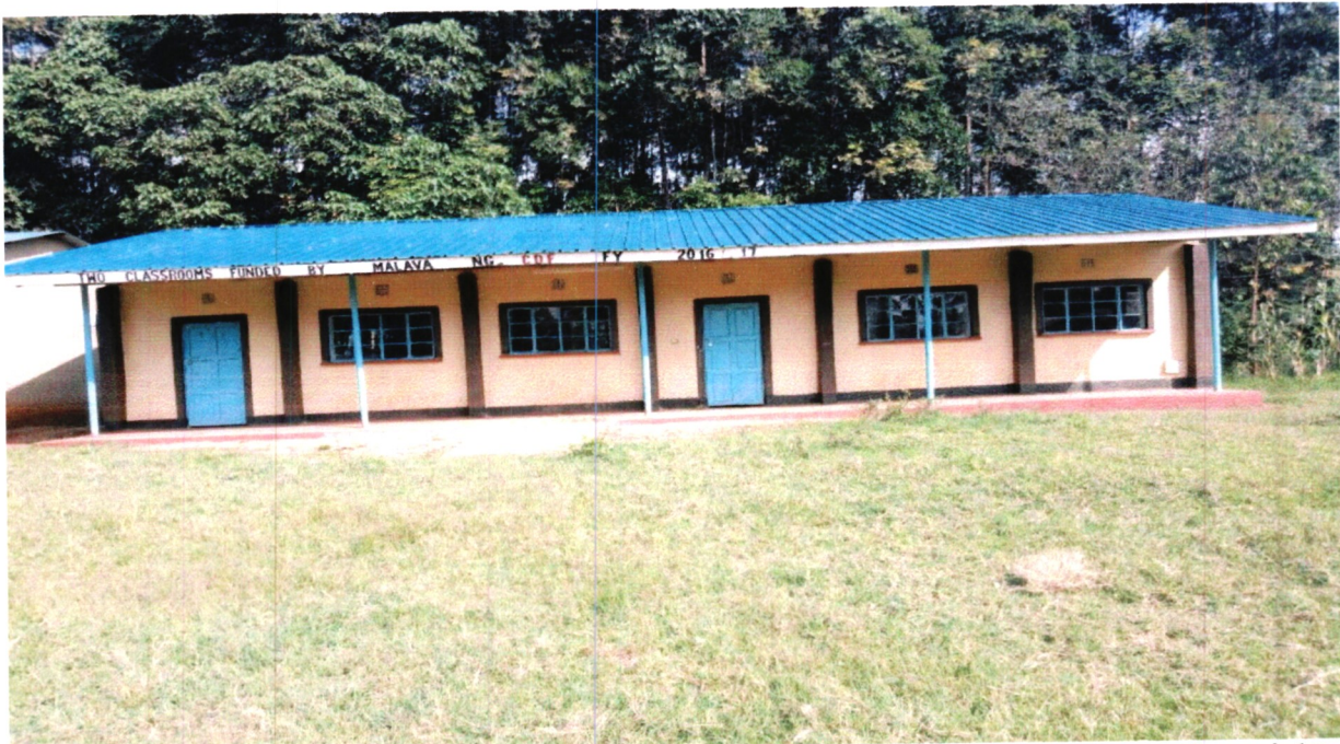
Shihome Primary School construction of 2 classrooms funded by Malava NGCDF Financial Year 2017/2018
