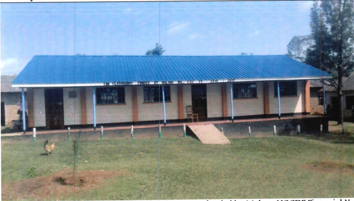
Lukume Primary School construction of 2 classrooms funded by Malava NGCDF Financial Year 2017/2018
