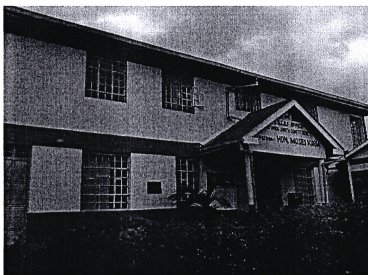
FIG1.2:The Renovated NGCDF Office in Gatundu South Constituency which was constructed 4years ago.
