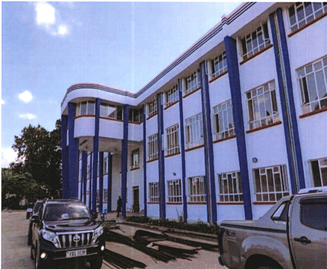
Picture 15: Karuri Health Centre new block that will house the additional outpatient wing, a 16-bed maternity ward, a 10-bed general ward, a pediatric ward, a laboratory, and a theatre.
