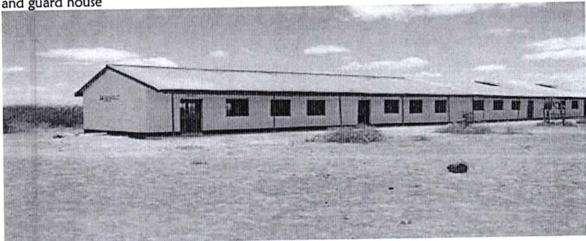
Beramo Primary School: Renovation of seven classrooms FY 2023/2024
