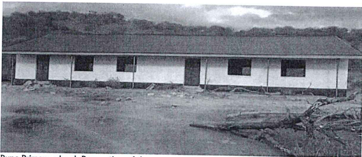
Buna Primary school: Renovation of classrooms
