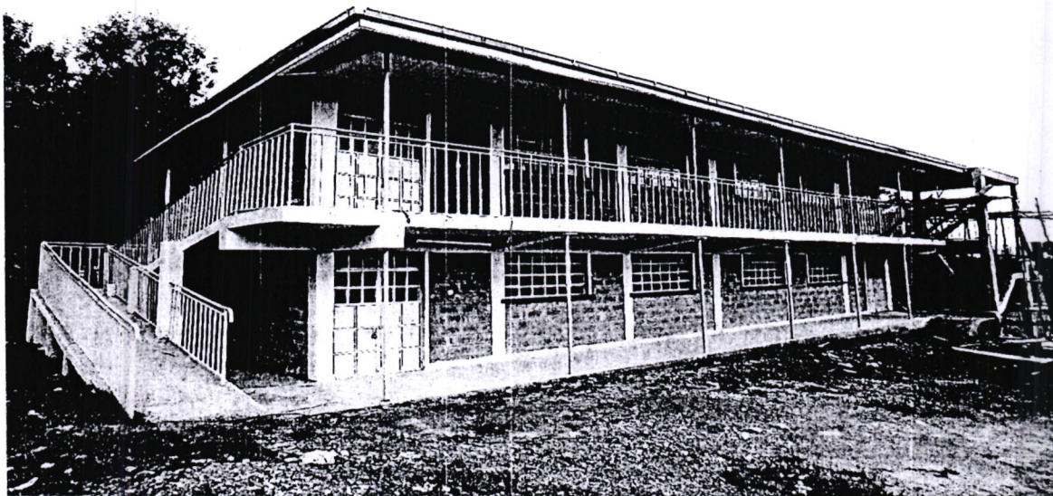
Completed 4no classrooms at St. Patricks mixed day secondary school
