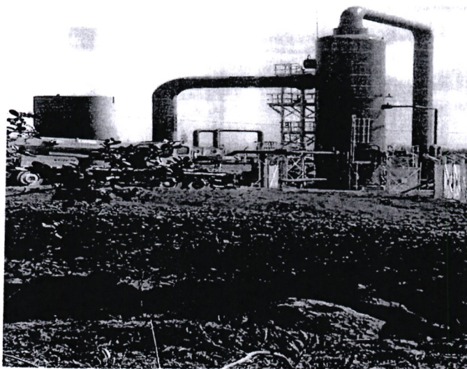
Steam Gathering System at Menengai Geothermal Field
