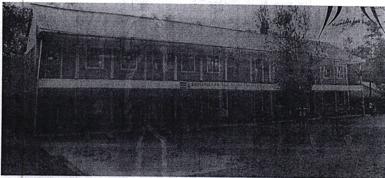
Ebuchinga Primary School –Construction of 8 No Classrooms Storey
