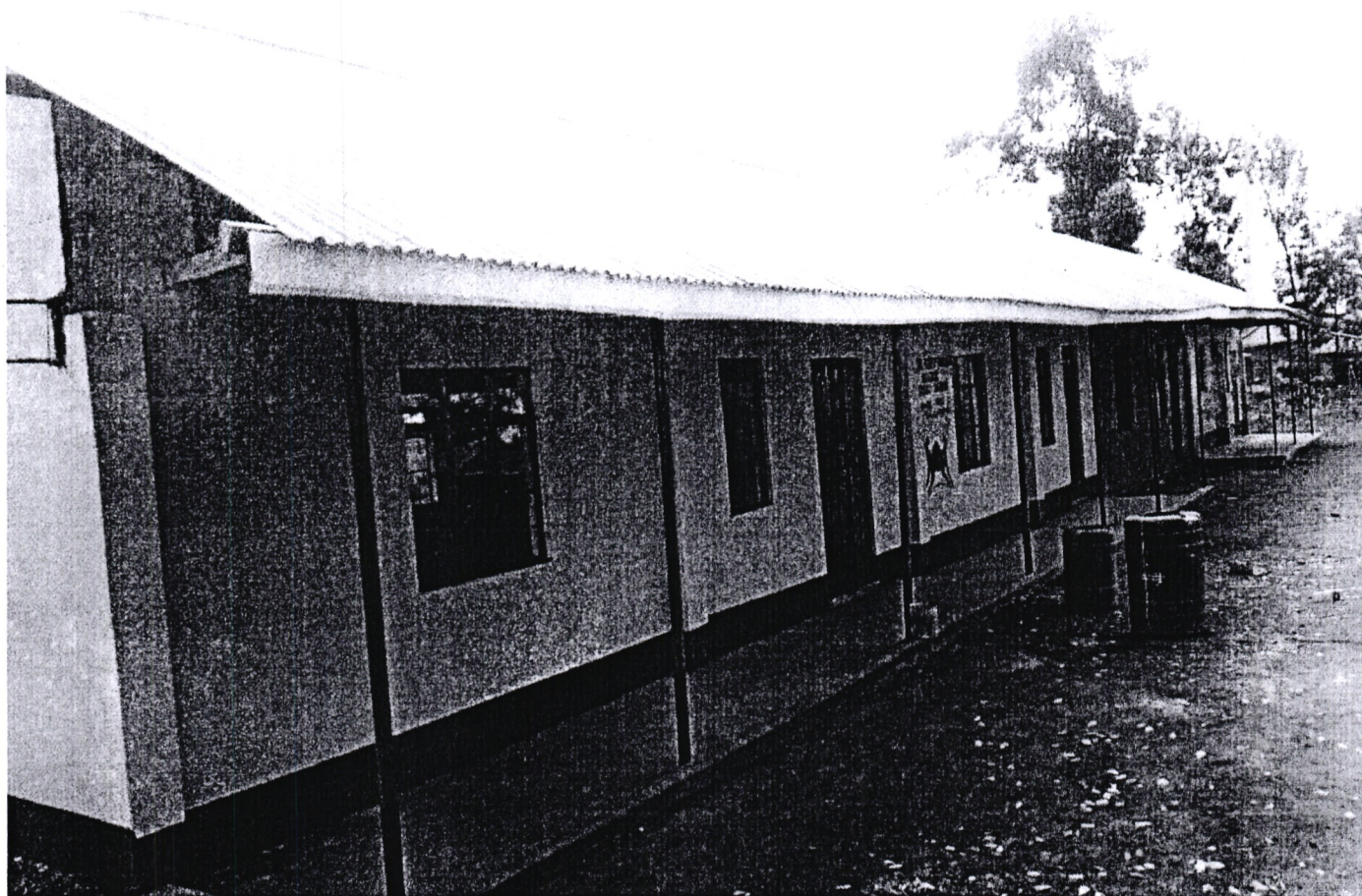
SENIOR CHIEF BARAZA PRIMARY SCHOOL CLASSROOMS RENOVATED BY SUNA WEST NGCDF
