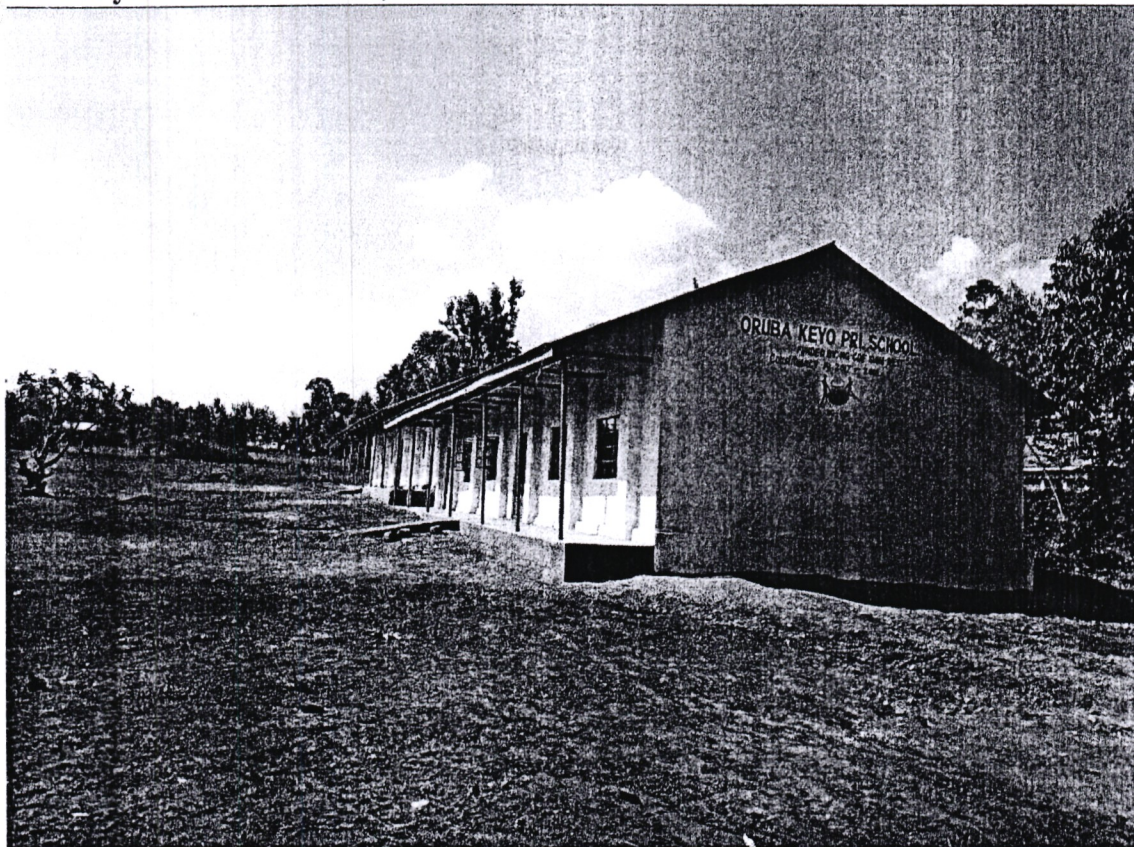
ORUBA KEYO PRIMARY SCHOOL. TWO NEW CLASSROOM CONSTRUCTED BY SUNA WEST NGCDF
