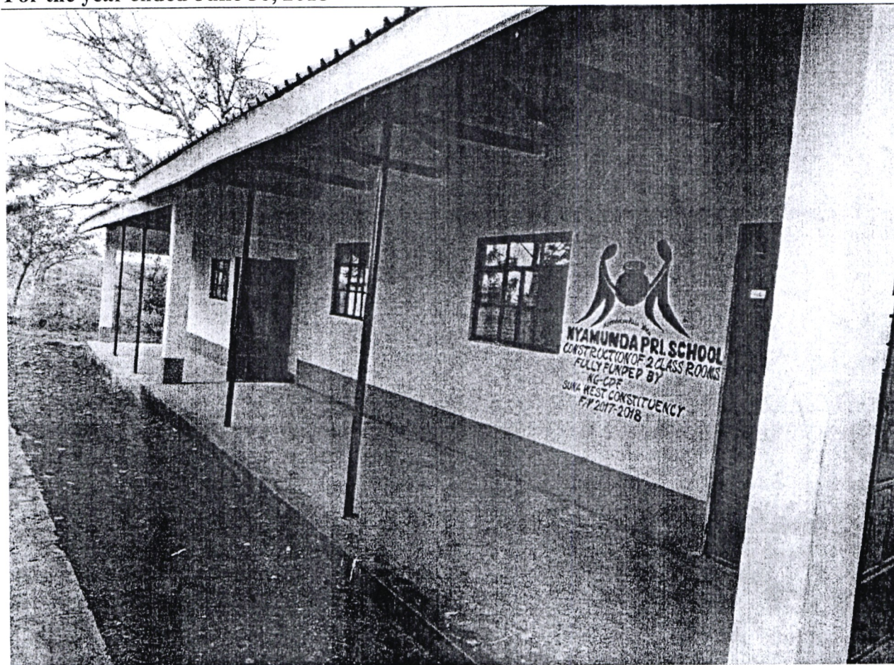
NYAMUNDA PRIMARY SCHOOL IN SUNA WEST NGCDF TWO NEW CLASSROOMS CONSTRUCTED
