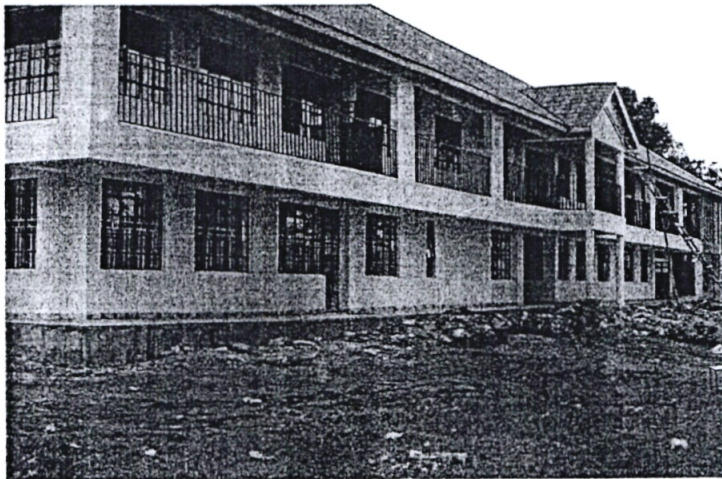
Kwa Secondary School. Construction of storey building 4 roomed Administration and 4classrooms.
