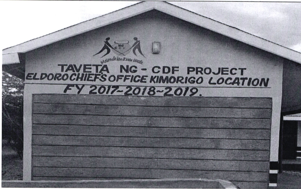
Complete construction of Eldoro Chiefs Office
