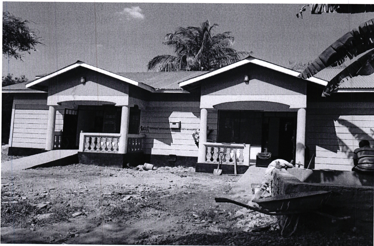
Construction of twin staff houses at kitobo secondary school
