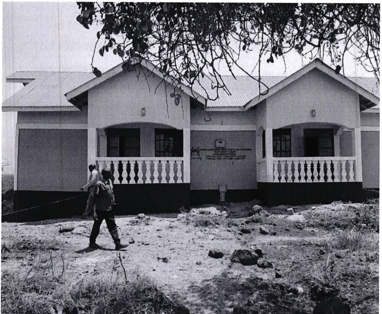
Lumi secondary school- construction of twin staff houses project
